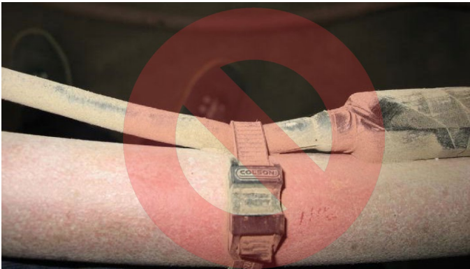
Figure 23. Do not use Zip-Ties Directly on Cables
