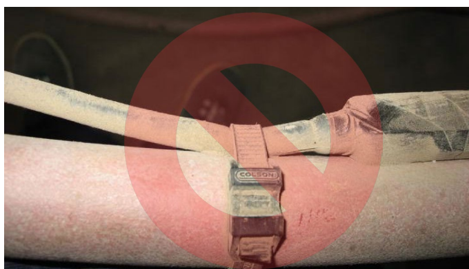
Figure 24. Do not use Zip-Ties Directly on Cables
