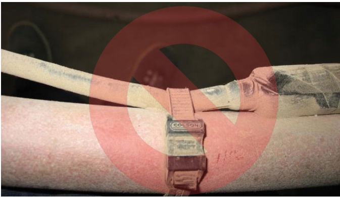
Figure 45. Do not use Zip-Ties Directly on Cables
