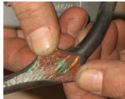
Figure 6. Do not use Zip-Ties Directly on Cables
