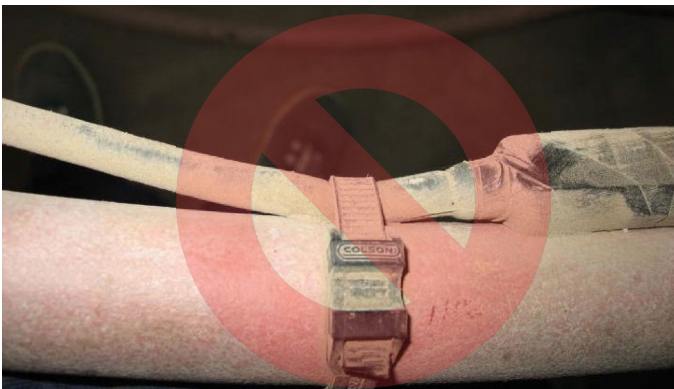
Figure 17. Do not use Zip-Ties Directly on Cables
