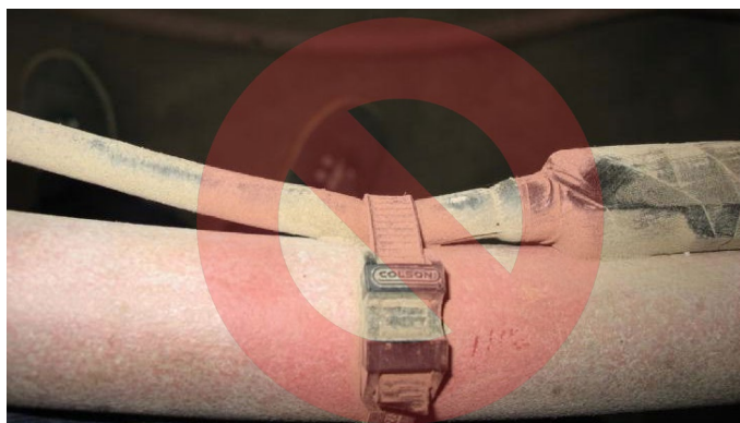
Figure 25. Do not use Zip-Ties Directly on Cables
