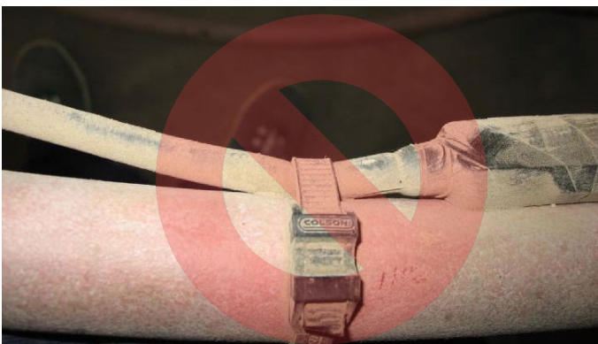
Figure 24. Do not use Zip-Ties Directly on Cables
