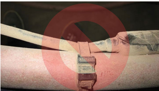
Figure 9. Do not use Zip-Ties Directly on Cables
