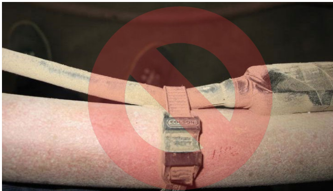
Figure 6. Do not use Zip-Ties Directly on Cables
