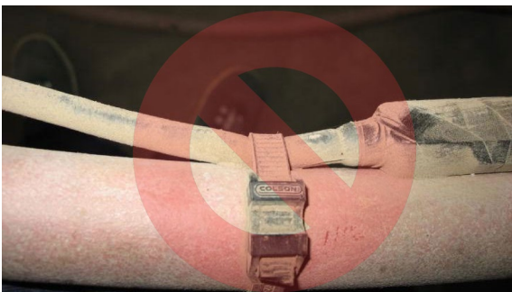
Figure 10. Do not use Zip-Ties Directly on Cables
