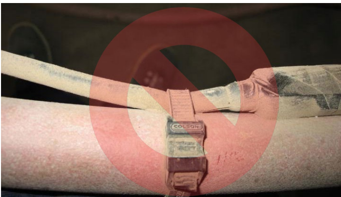
Figure 24. Do not use Zip-Ties Directly on Cables
