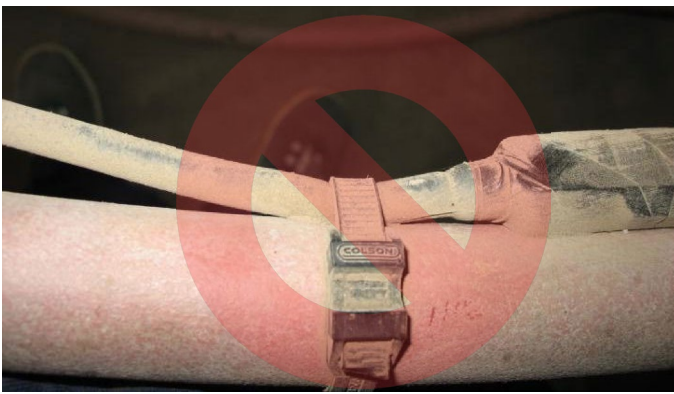
Figure 6. Do not use Zip-Ties Directly on Cables
