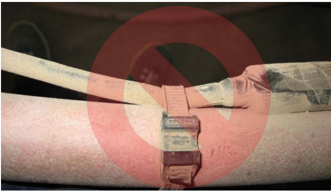
Figure 45. Do not use Zip-Ties Directly on Cables
