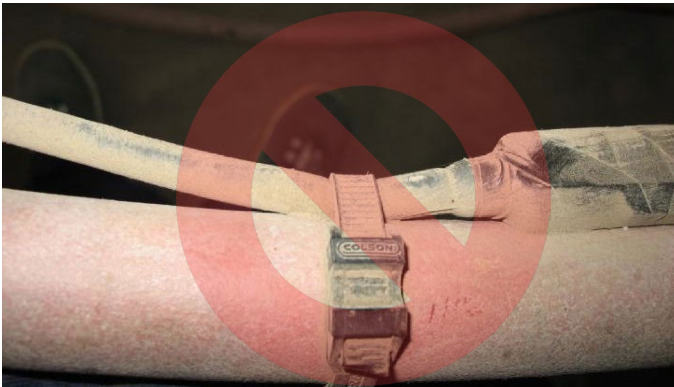
Figure 14. Do not use Zip-Ties Directly on Cables
