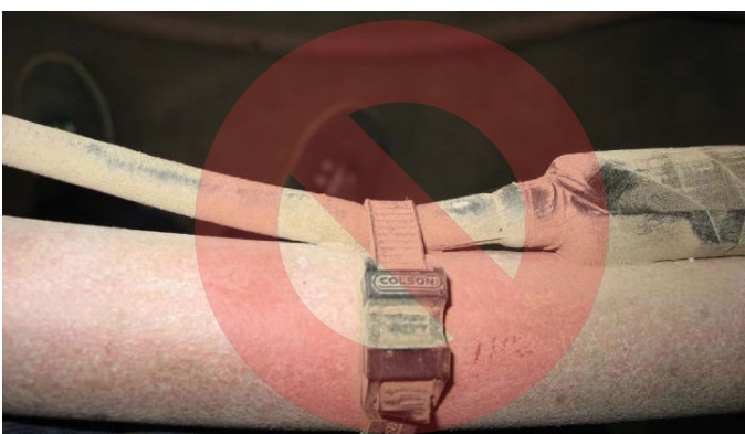
Figure 11. Do not use Zip-Ties Directly on Cables
