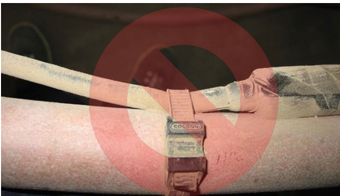
Figure 16. Do not use Zip-Ties Directly on Cables
